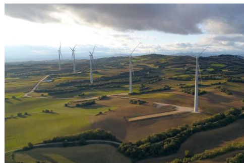
Wind farm in Navarra (Spain)
